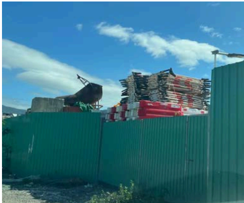
Application area filled with plastic fences (Application No. A/YL-KTN/889, photo taken on 29/05/2024)
