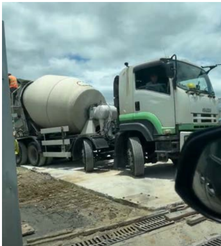
Application area with a cement mixer truck (Application No. A/YL-KTN/775, photo taken on 29/05/2024)
