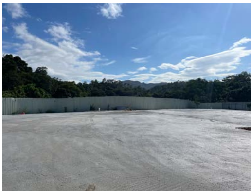
Concrete land without structures (Application No. A/YL-TT/573, photo taken on 29/05/2024)
