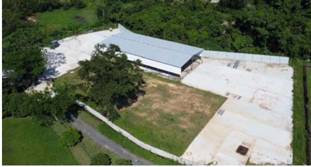
(Application No. A/YL-KTN/885, photo taken on 29/05/2024)
